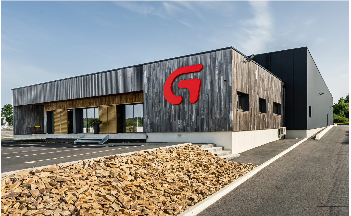
Poplar THT cladding - Gauthier transports
