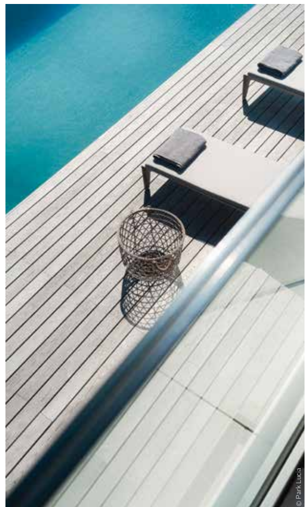
Casa Park Lucia - Ash decking THT, B-Fix® invisible fixing
