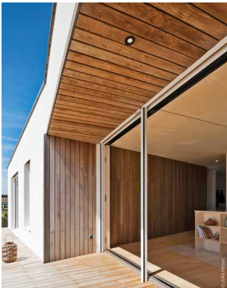
Thermo treated Ash Cladding - Emeline Poulain Architect
